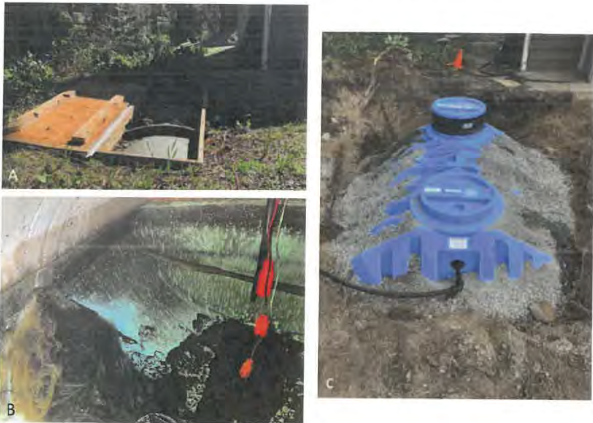
Figure 2. Water storage tank before (A, B) and after (C) replacement.
